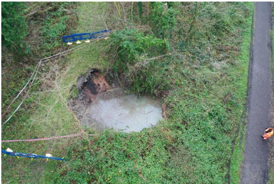
Figure 2: A clay shaft which collapsed in December 2023.
