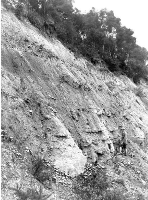
Figure 3: The backscarp of the Lloyds landslip.
